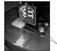
Remove cover off motor terminal box.
